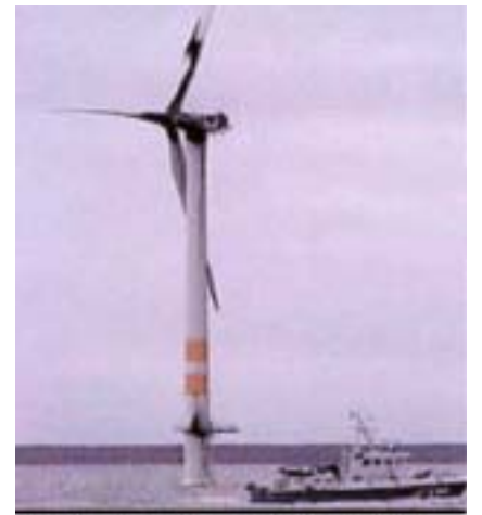
Turbine fire in nacelle burns itself out, thought to be caused by overheated parts igniting wire insulation. Newer turbines have fire suppression equipment to contain and extinguish fires within the structure.
